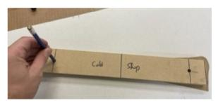
4. Use small drill bit to drill both holes through template to ensure accuracy. Then remove template and use 1/2" drill bit to enlarge hole for toggle anchor. (drill bits not included)
